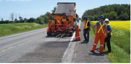
to get an emulsion and aggregate to blend, spray and apply cleanly and quickly. It is a type of Macadam which is created to fill holes or repair imperfections to asphalt or concrete pavements. The product can also be used to stabilize shoulder wear and erosion or surface, treat driveways and other areas."
